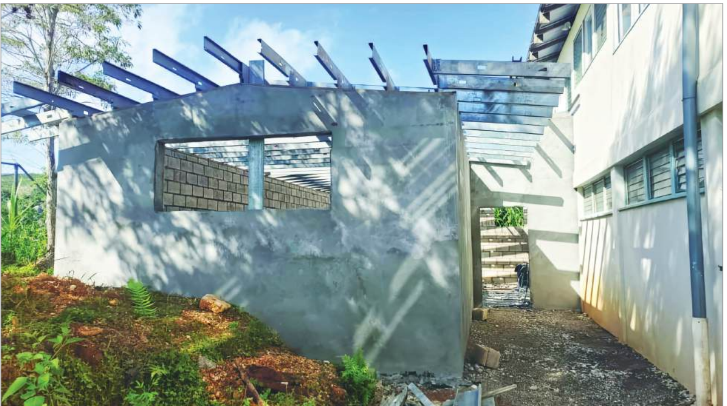
Construction of the surgical center
