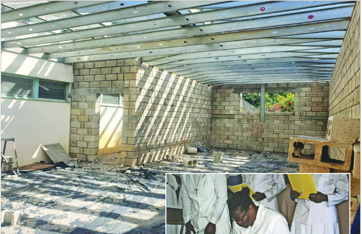
Construction of the surgical center
